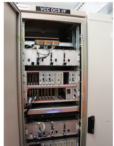
A temporary control centre at Old Dalby (left) is linked to a signal equipment room housing the System Management Centre and the Vehicle Control Centre which provides the core interlocking functions (right).
